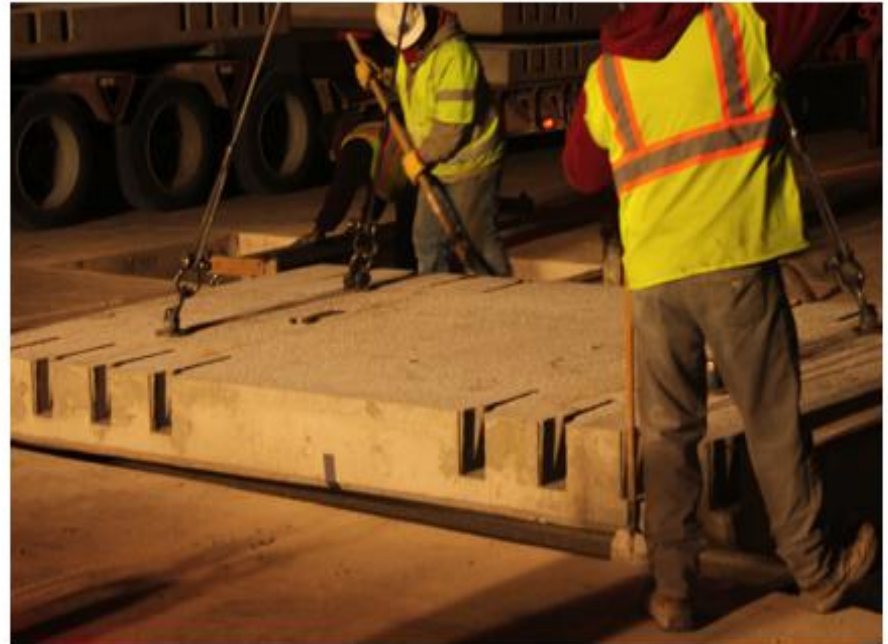
Precast pavement creates a full-depth repair of the roadway with minimal closures of the busy I-294 corridor. Photo Courtesy of Utility Concrete.
